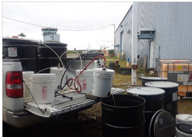
Exhibit 2-5: Filtering MW development water through portable GAC filtration system.
