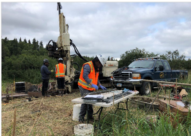
Exhibit 2-2: Geologist James Dutt logging a soil boring during drilling at AKNPW-204.
